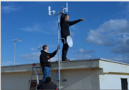
Fig. 2. People installing a CN node on the roof of a building (source: https://blog.ninux.org ).
